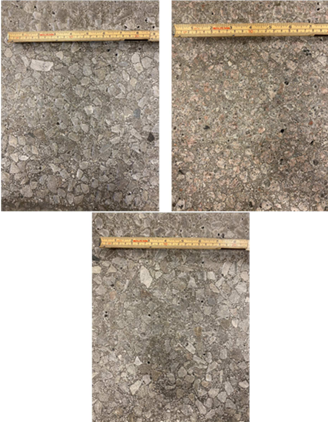
Figure 150. Example of slabs surface.
